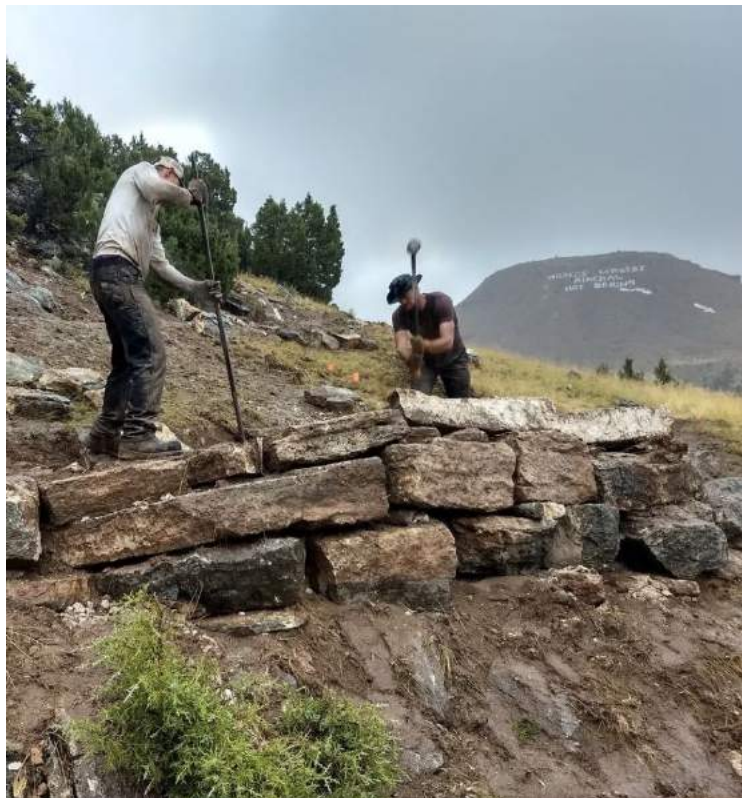
Workers build retaining wall on T Hill Trail (2019)
